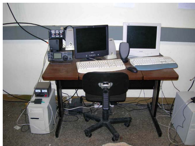
Communications system with integrated computer control, tracking system, and antenna pointing control.
