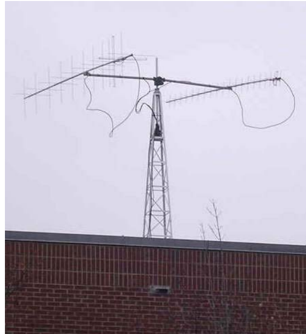
PANSAT communications tower with 432 and 140MHz circularly polarized antennas on top of the ECE Building.
